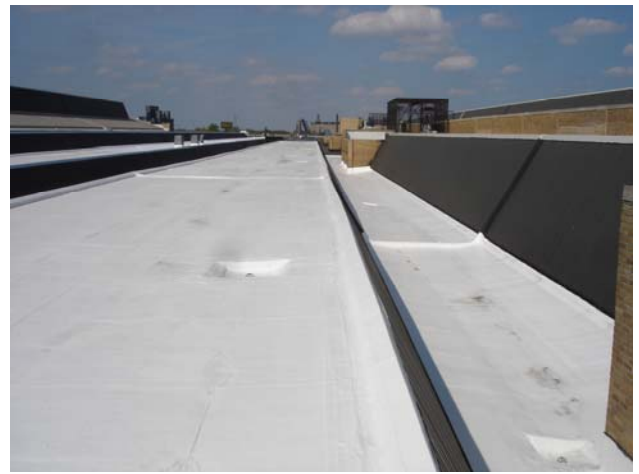
After - a reflective, white Roof-Tek ® SSP system was applied
