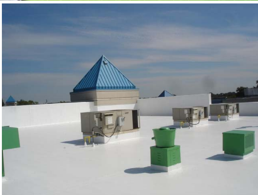
Completed and restored SSP roof project
