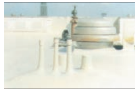
Polyurethane spray foam is self flashing on penetrations and walls.
