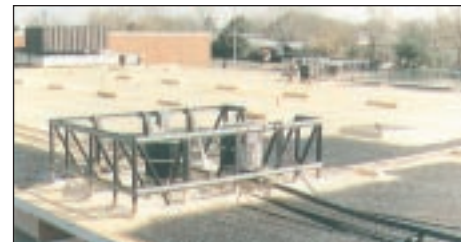
Polyurethane spray foam is especially suited to complex roofs.
