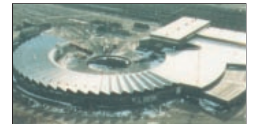
A Minnesota roundhouse is insulated and protected by BaySystems spray foam.
