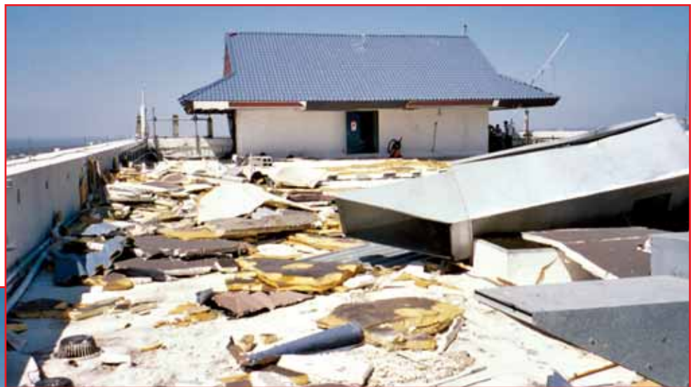
Photos 1 and 2 – Impact of reduced fastening patterns.
