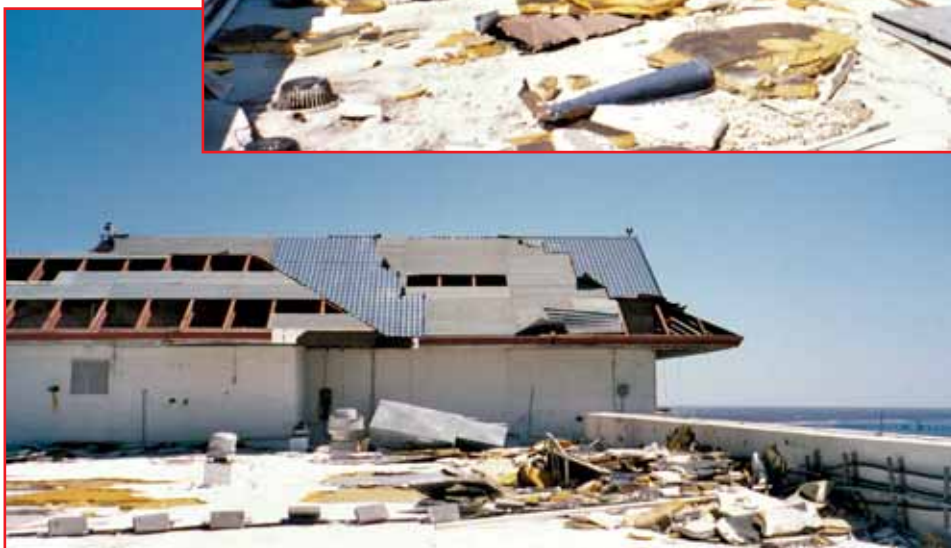
Photos 1 and 2 – Impact of reduced fastening patterns.
