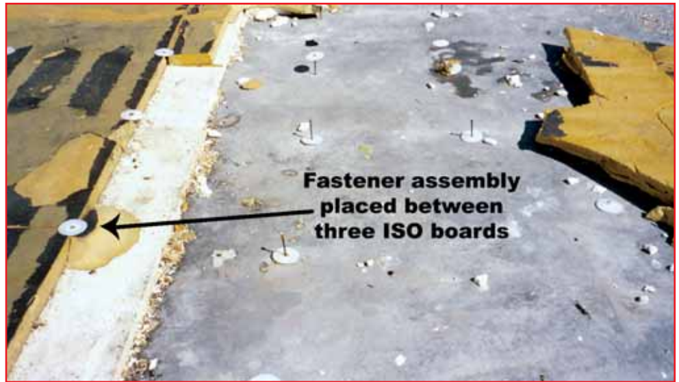
Photo 5 – Fasteners were driven between ISO sheets, shared by adjacent boards.
